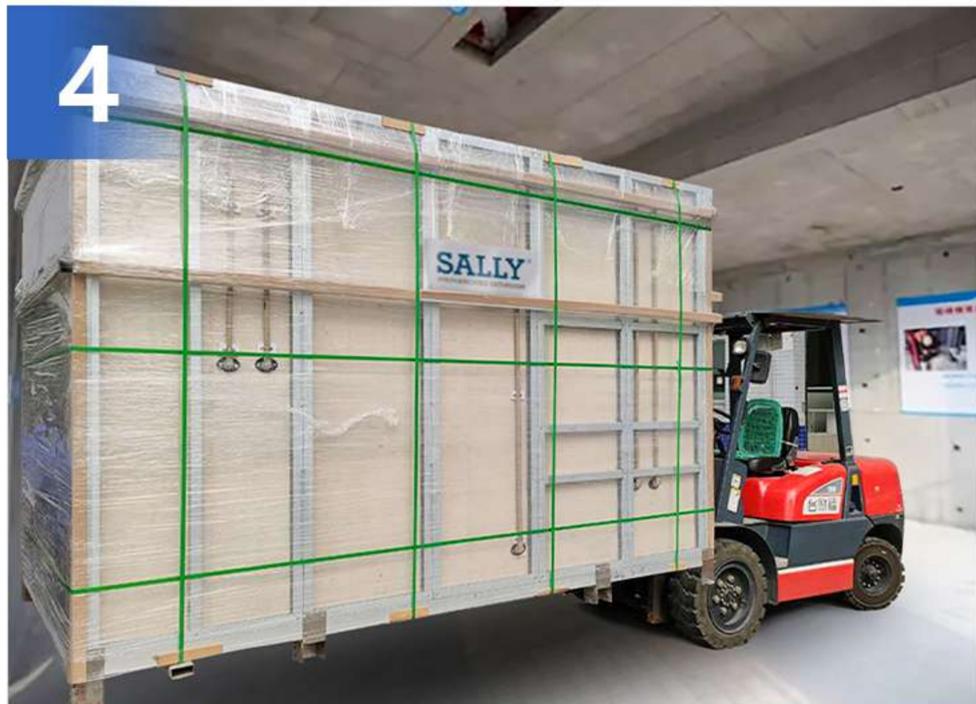
4 POD MOVED INTO POSITION VIA
