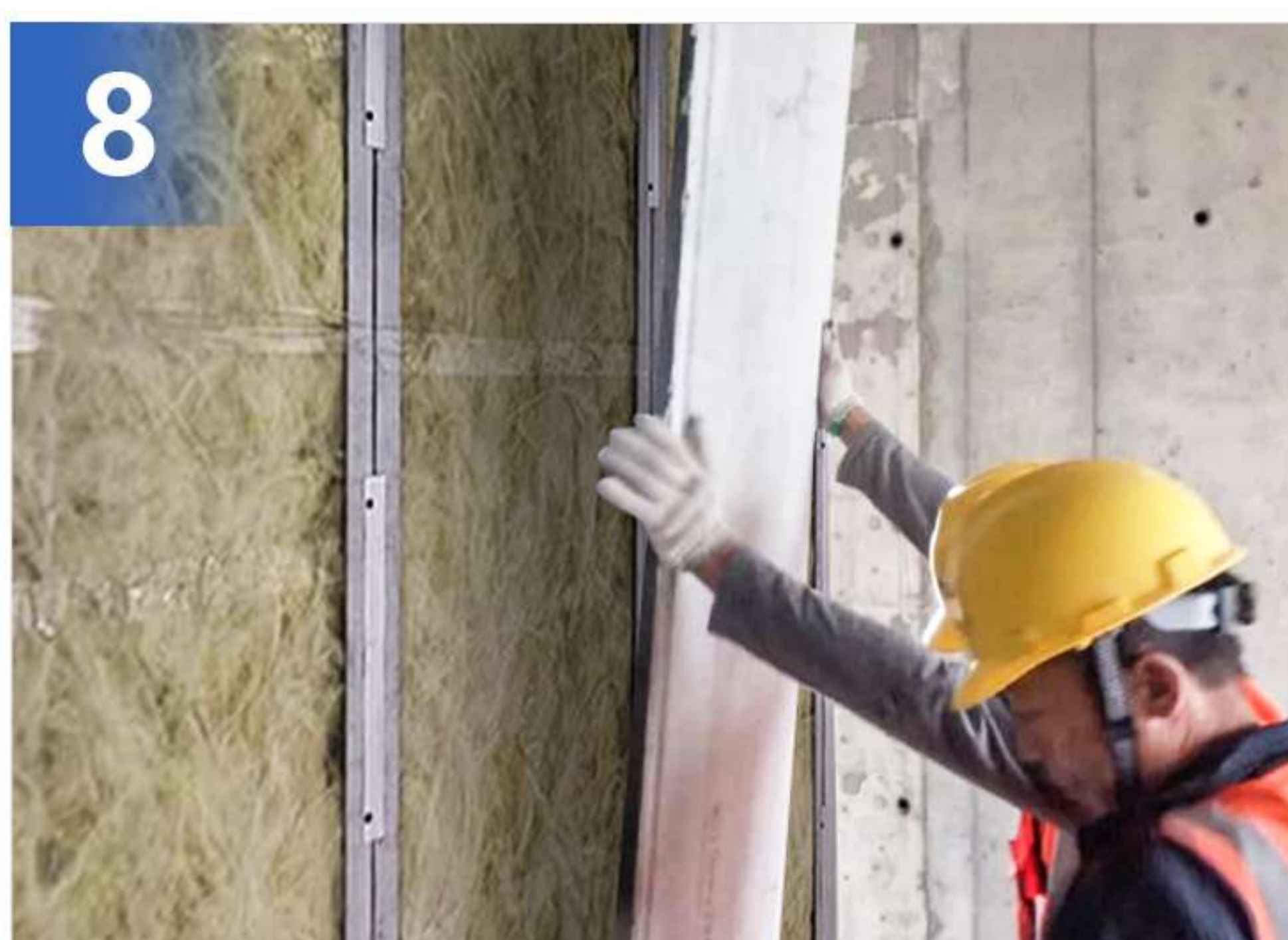
8 EXTERIOR SHEETED WITH PLASTERBOARD
