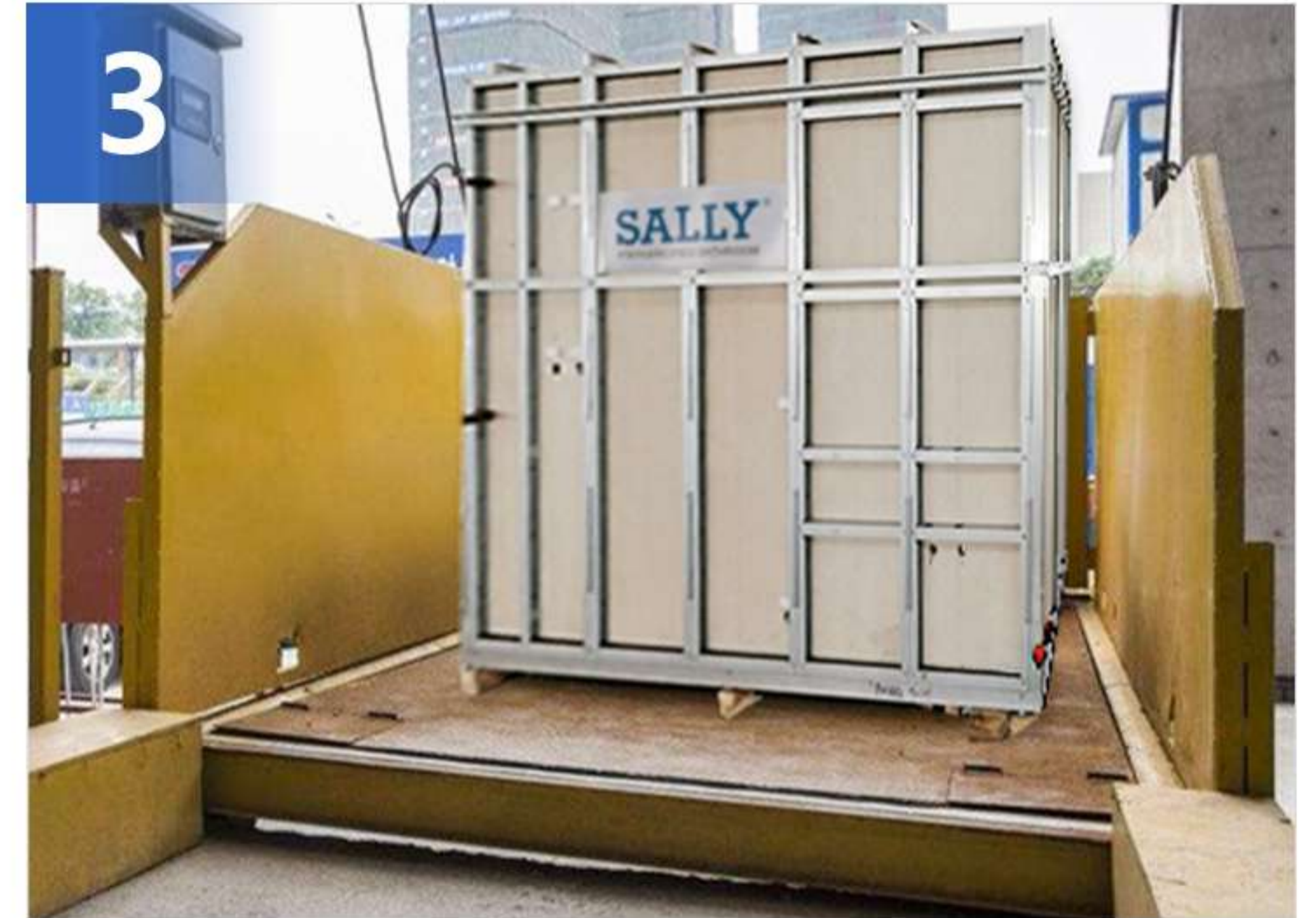
3 POD LANDING ON PLATFORM
