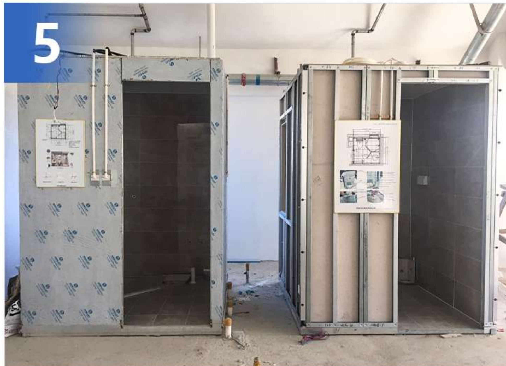
5 POD PLACED AND UNWRAPPED
