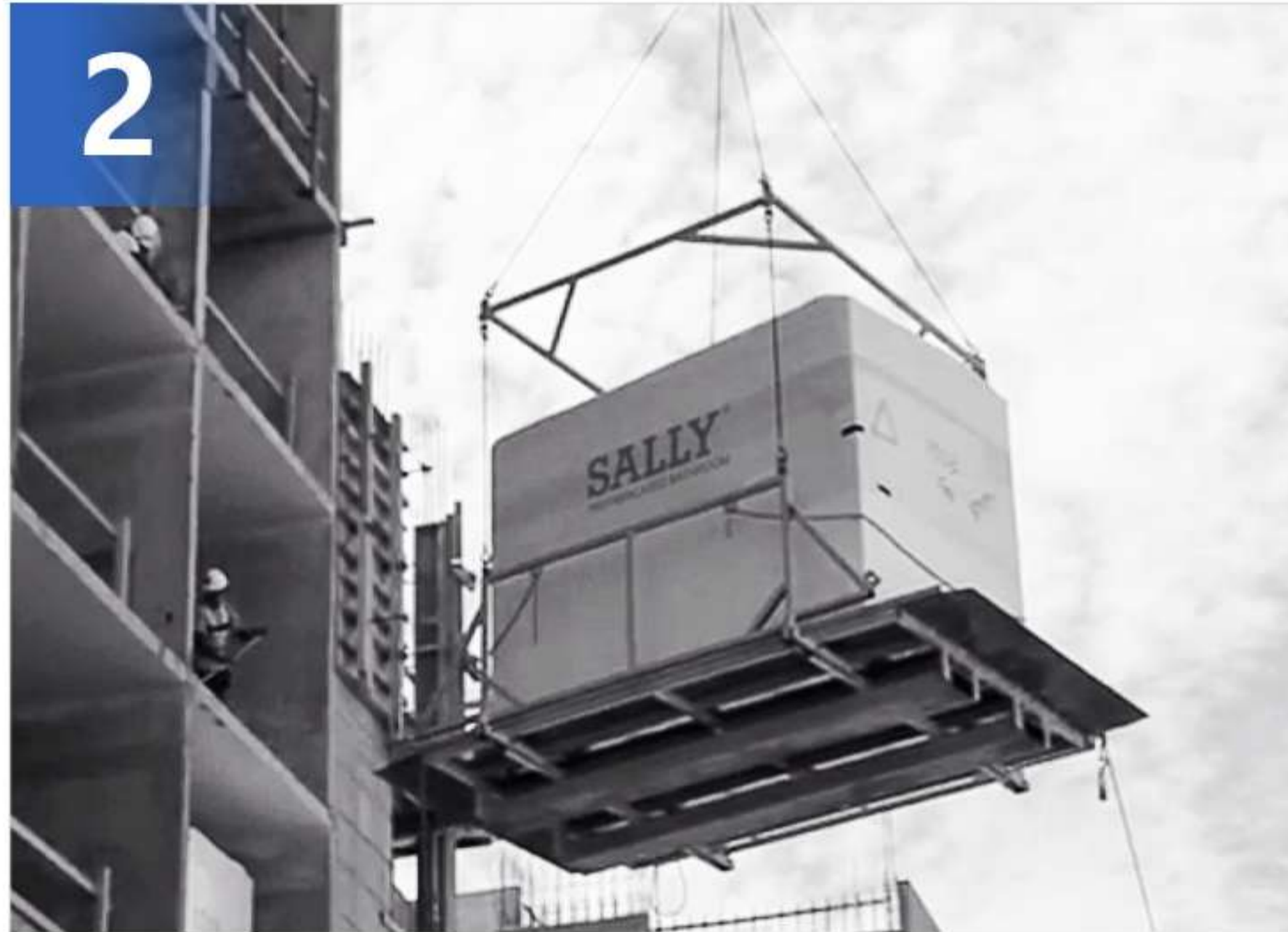
2 POD LIFTED VIA CRANE
